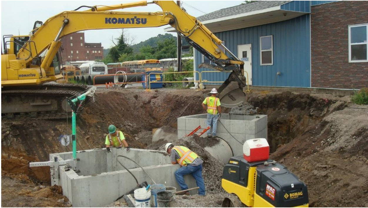
We placed concrete to house 66-inch reinforced concrete pipe structures.
